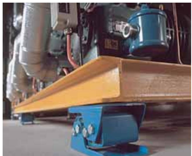
Cooling compressors on type ESL mounts
